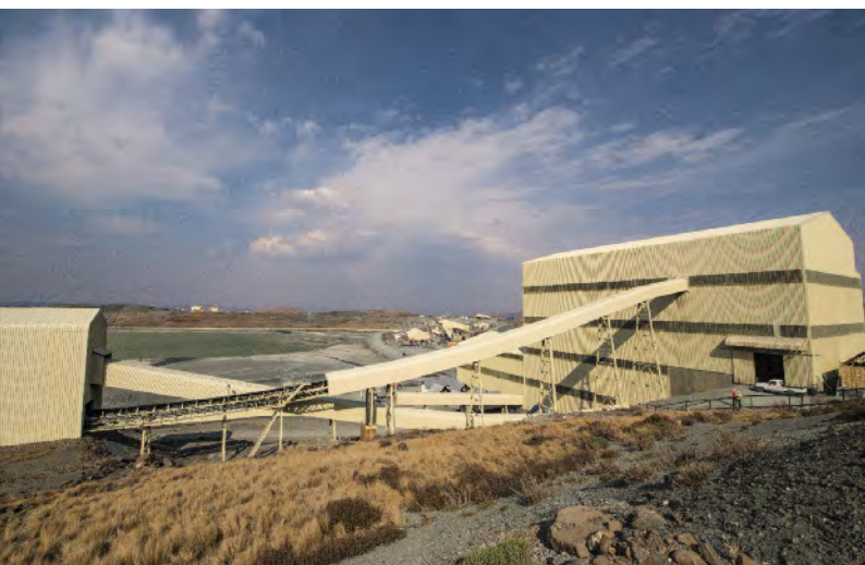
Figure 12. This state-of-the-art processing plant at Letšeng is designed to minimize damage to large diamonds and improve the recovery rate. The plant takes advantage of the region's mountainous topography by incorporating a gravity-fed recovery process. Photo by Robert Weldon/GIA.
