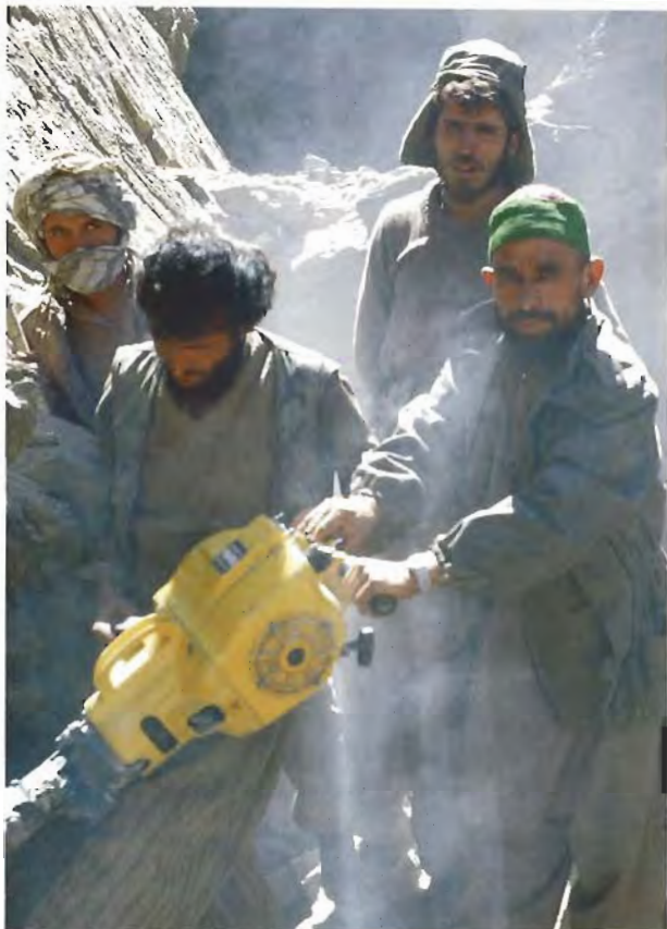
Figure 8. Diesel-powered drills are also used to remove the hard wallrock. Because the miners wear virtually no protective gear, injuries from falling or flying rock—as well as illness from the carbon monoxide fumes—are common. Photo by Gary Bowersox.
