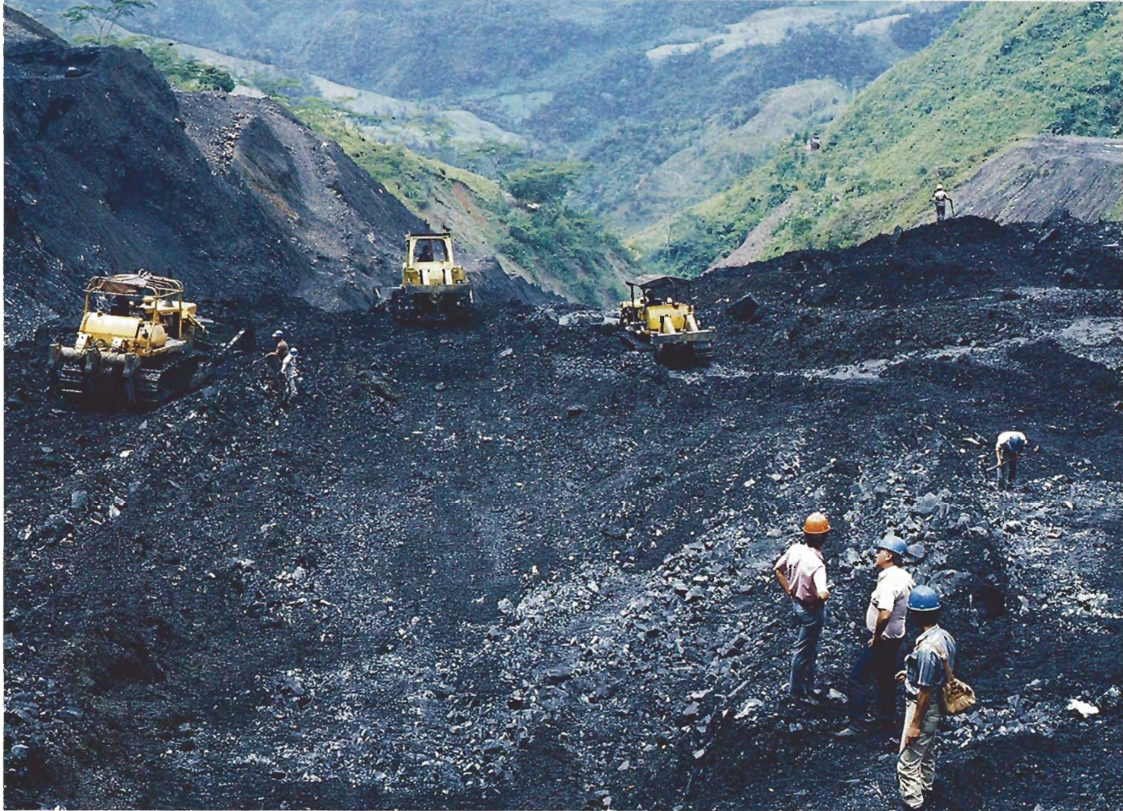
Figure 6. Today, the mine owners at Coscuez use bulldozers to retrieve the emeralds more quickly and efficiently by the open-cut method. The bulldozers clear layers of black shale until the potentially emerald-bearing veins of white calcite are uncovered. On the right, a lone miner searches the white calcite for emeralds. Photo by Jack Rotlewicz.
